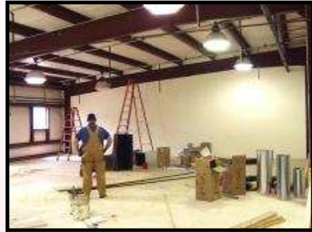
Mezzanine Work In Progress
